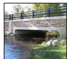
Figure 4: Three-sided box bridge
