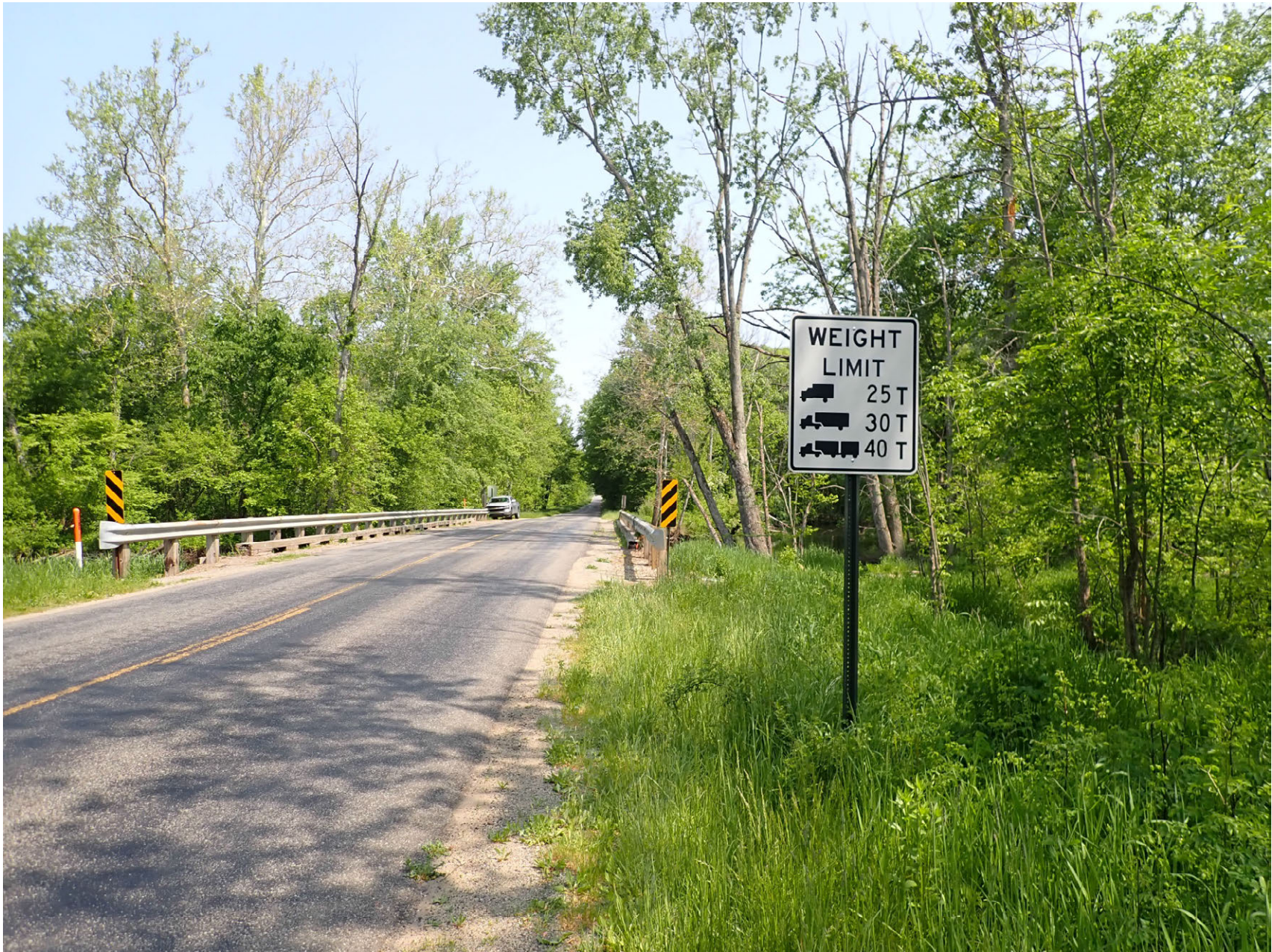
Posting sign, looking north
