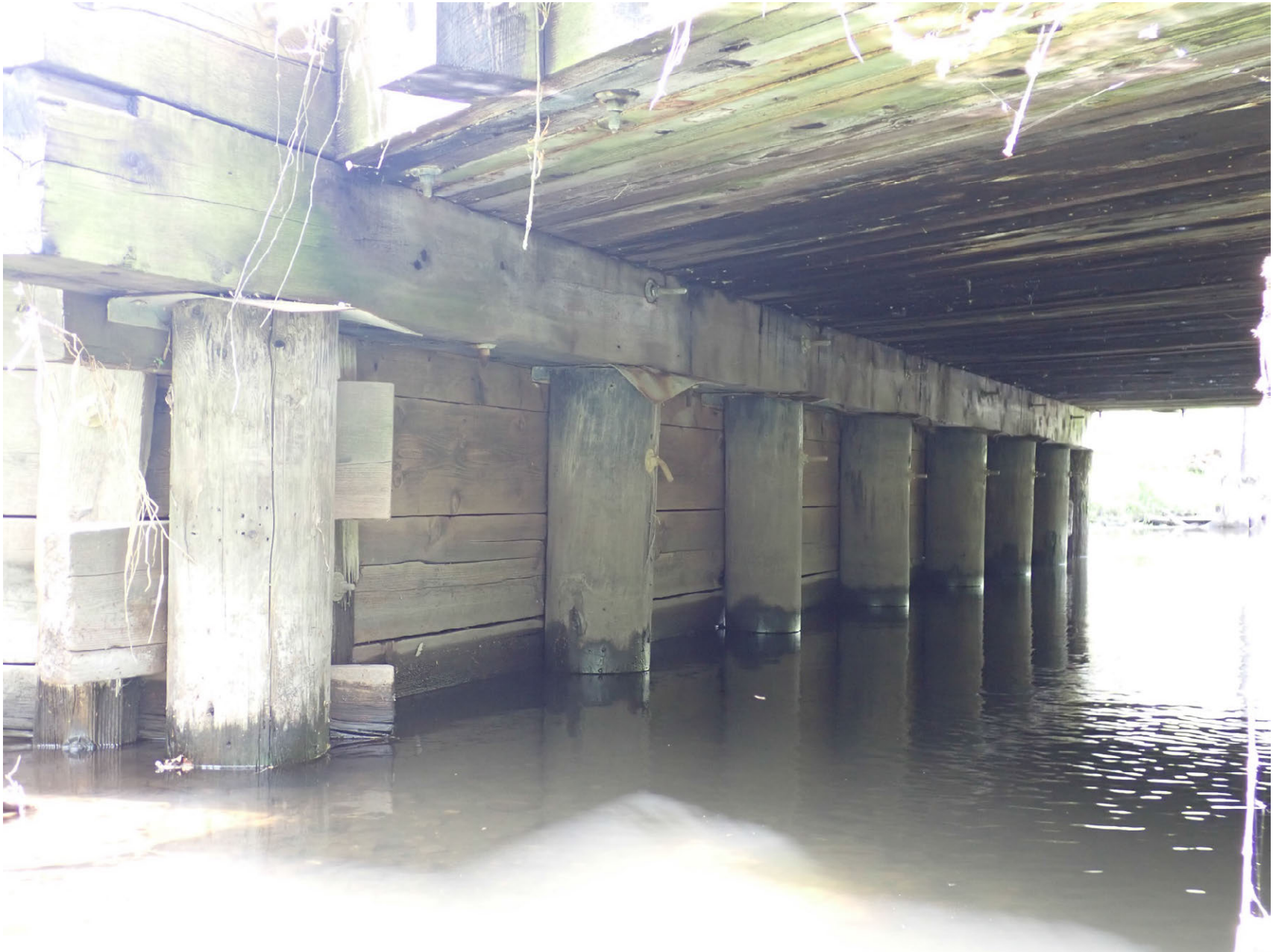
South abutment elevation
