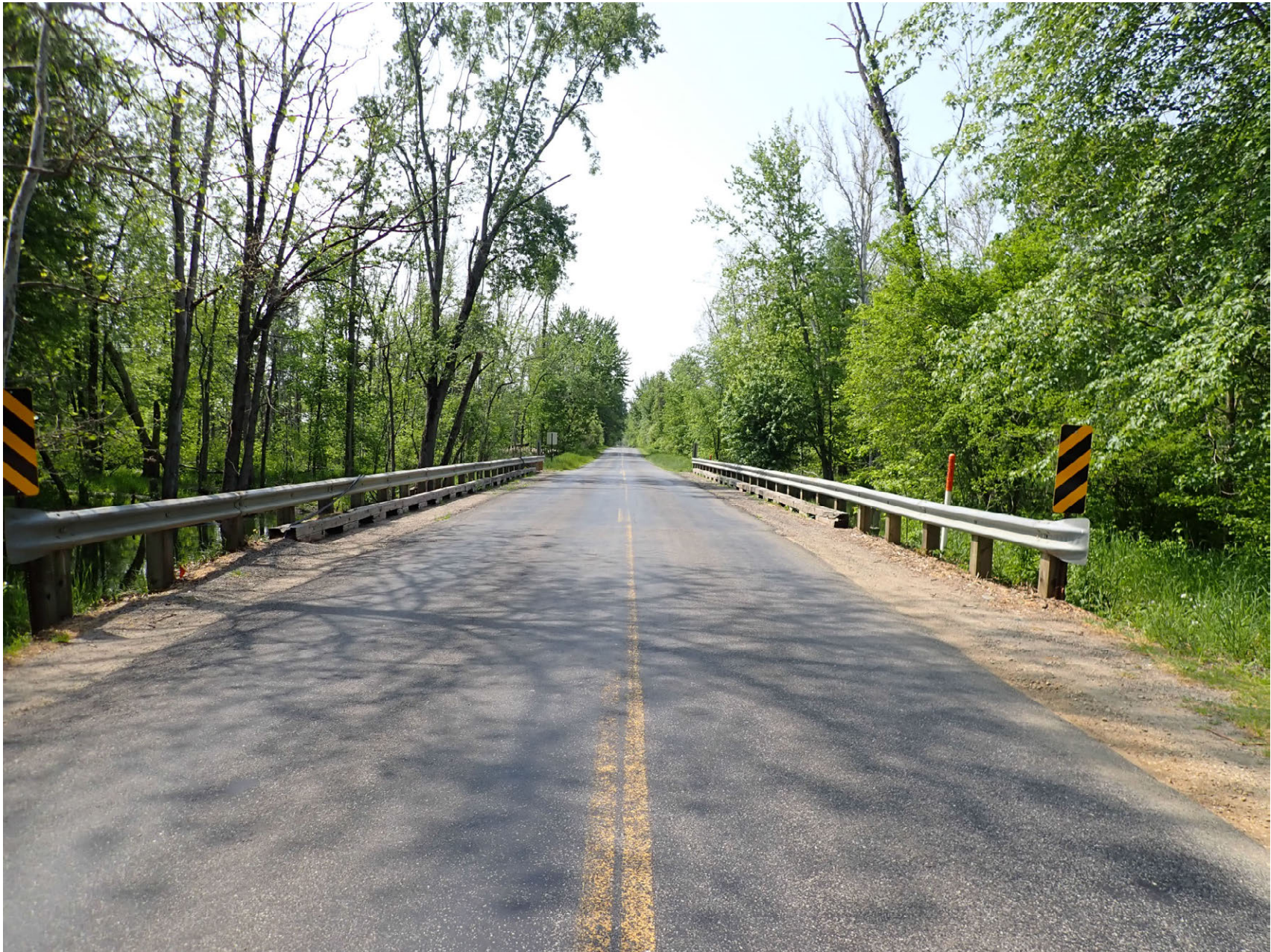
Bridge section, looking south
